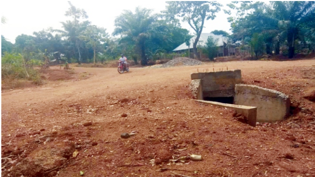
Newly constructed drainage system in Ndifu Alike community in Ebonyi State
