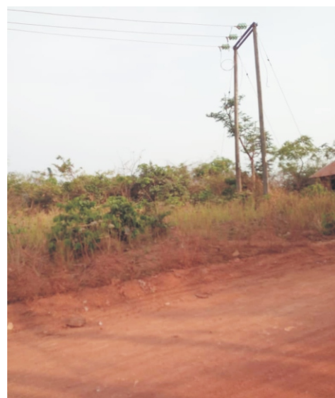
Royal Salt ongoing Rural Electrification in Ndifu Alike community, Ebonyi State
