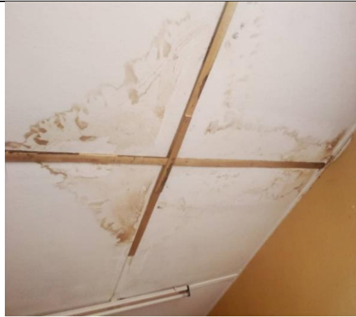
Repaired a Leaking Roof at their Facility
