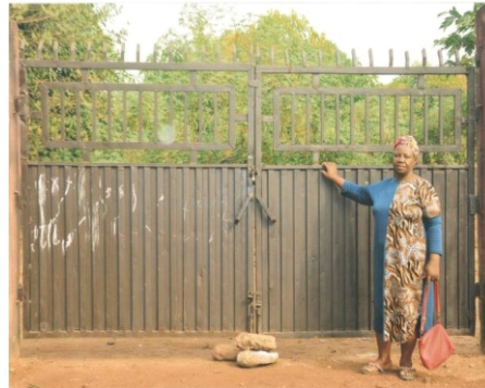
Provided Security Gate at the Entrance Health facility
