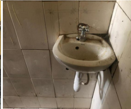
Used to renovate the Pipe of the Wash Hand Sink
