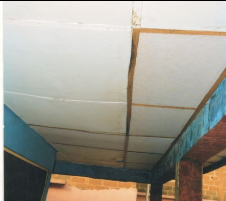
Repairs of Facility Ceiling Board
