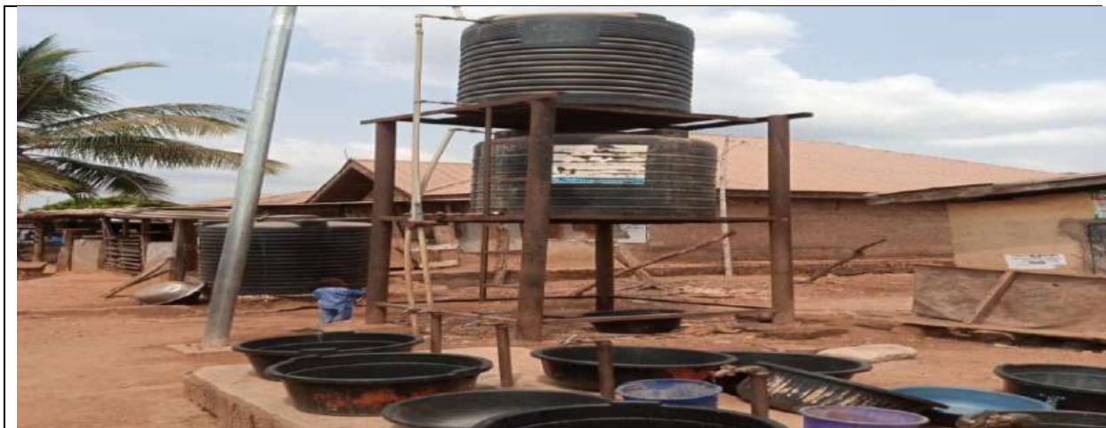
Borehole project delivered in Udugborevo Quarters in Ikpeshi
