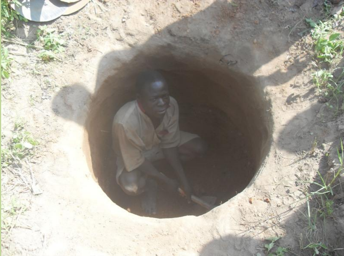
Pix: shows a Community member digging his toilet in Kuyizhi Community, FCT.
